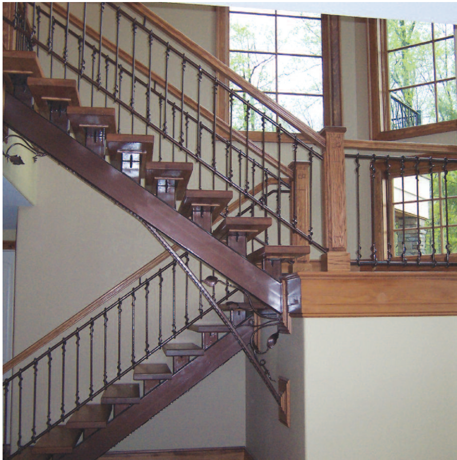
ABOVE: This mono string staircase was designed for a contemporary home with an outdoor fountain that begins in the front yard, runs indoors into the living room, and then out into the back yard. The client wanted the area to feel open, with nature-like elements.
