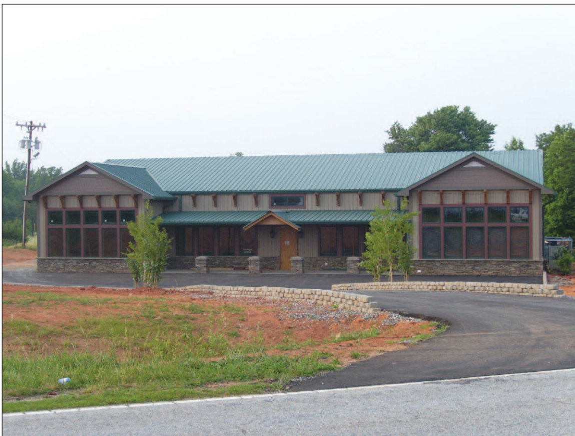
Heirloom Stair and Iron's new building is pictured under construction.
